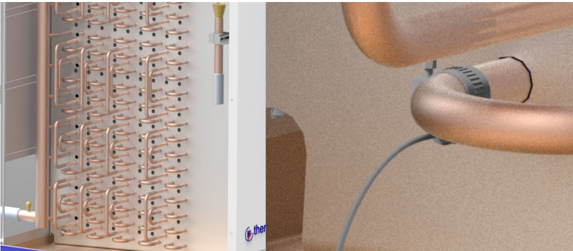
Figure 11: position sensor 1; case dry expansion
